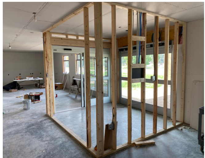
Entryway into building
