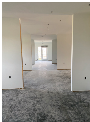
This photo shows the exam room hallway, where modular walls and doors will be installed to close off each room.
