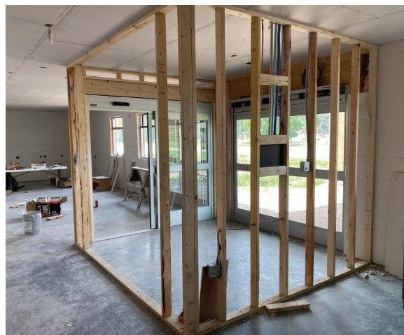
This photo shows where guests will enter the building and turn right toward the registration desk.
